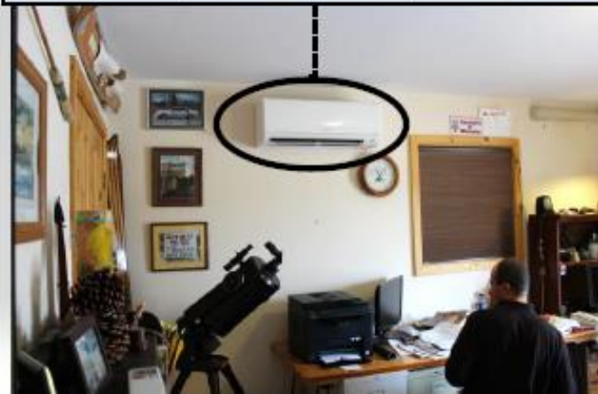
Indoor Cassette Unit (heat delivery) OFFICE Mitsubishi 9,000 BTU (0.75 ton)
