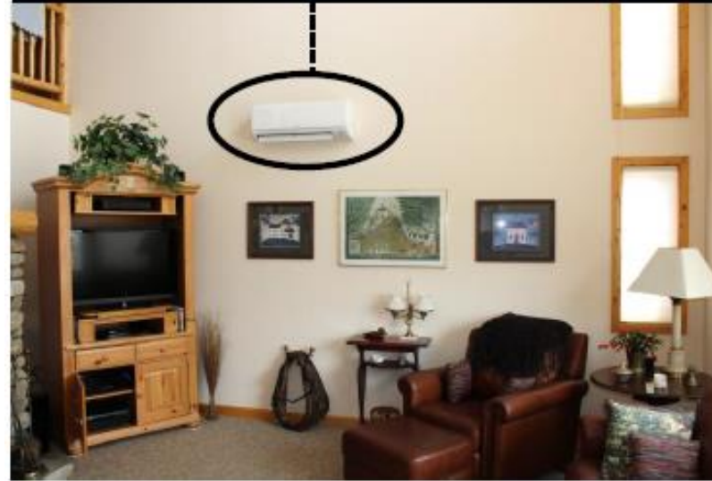
Indoor Cassette Unit (heat delivery) OFFICE Mitsubishi 9,000 BTU (0.75 ton)
